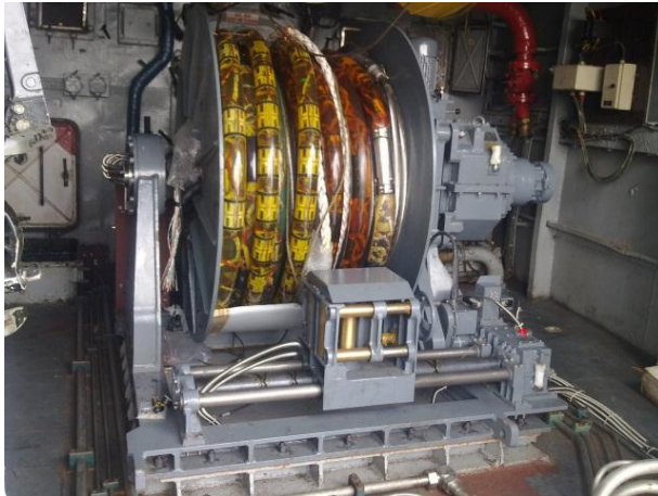
Fig.2. Cable and Array wound on Winch
