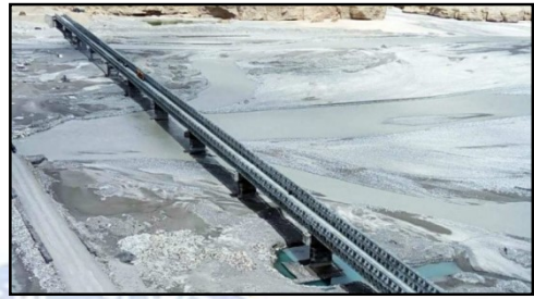
A road bridge built by India between Durbuk and Daulat Beg Oldi in eastern Ladakh | Representational Image | ANI
