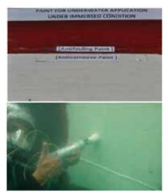
Anti-corrosive and anti-fouling paint application under immersed condition
