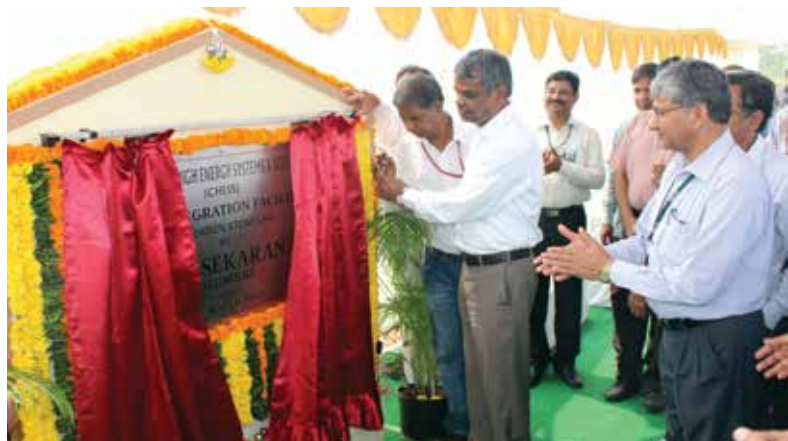
Dr VG Sekaran, DG (MSS) laying the foundation stone of HEL Integration Facility
