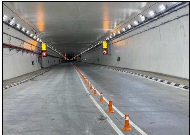
Rohtang Tunnel | Photo Credit: IANS
