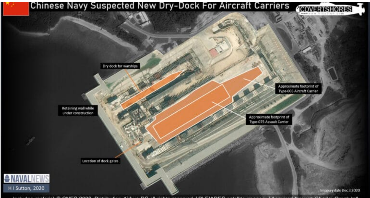
This recent satellite image shows how the new facility, believed to be a dry dock, will be large enough for China's new Aircraft Carriers
