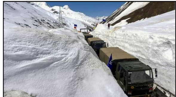
The BRO will ensure that Zoji La is blocked only 45 days instead of 95 days due to snow this winter.
