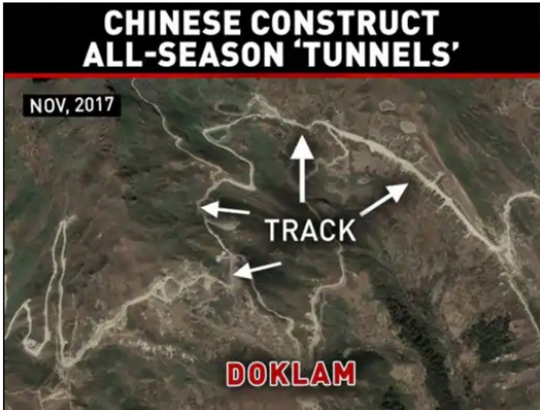
Since the 2017 India-China standoff, Beijing has tarred and reinforced its existing track in Doklam to make it an all-weather road. Courtesy: Google Earth
