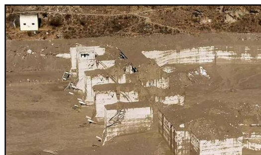
Chamoli: Damaged Dhauliganga hydropower project at Reni village, after a glacier broke off in Joshimath causing a massive flood in the Dhaul Ganga river, in Chamoli district of Uttarakhand, Sunday, Feb. 7, 2021 | PTI
