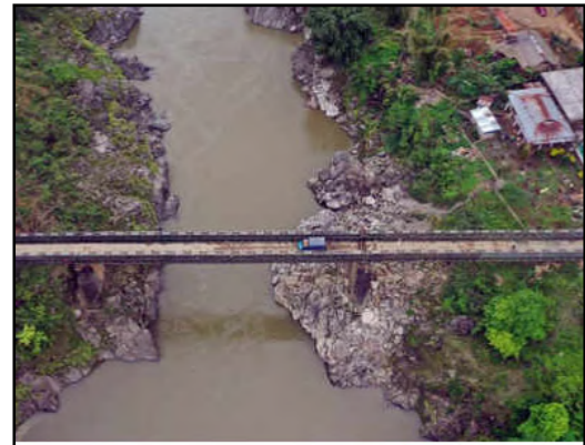
Daporijo bridge constructed by BRO
