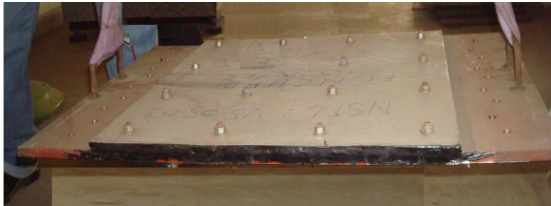
3 layer VDC applied on base structure
