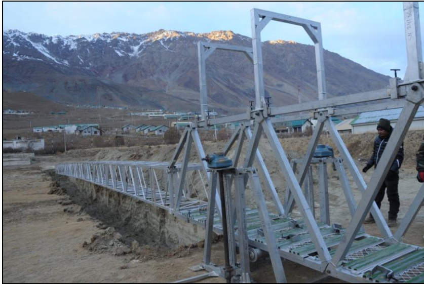
Launching of Mountain Footbridge
