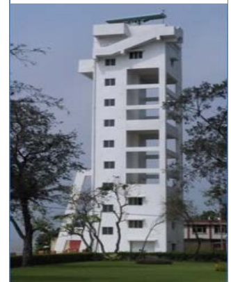
CSR installed in East Coast
