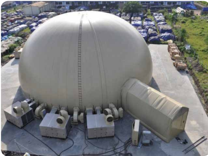
Air supported inflatable radome
