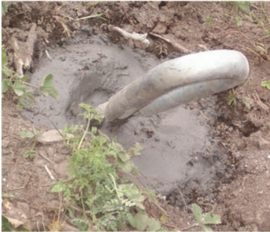
Anchor Pile Foundation
