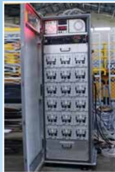
Sonar Cabinet using 16 n2 (and 2 spares) Nos of Power Amplifiers
