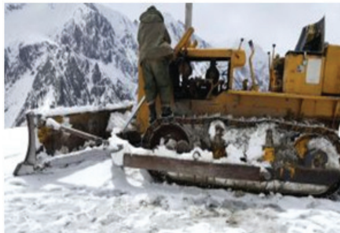
Angling of dozer blade for snow clearance
