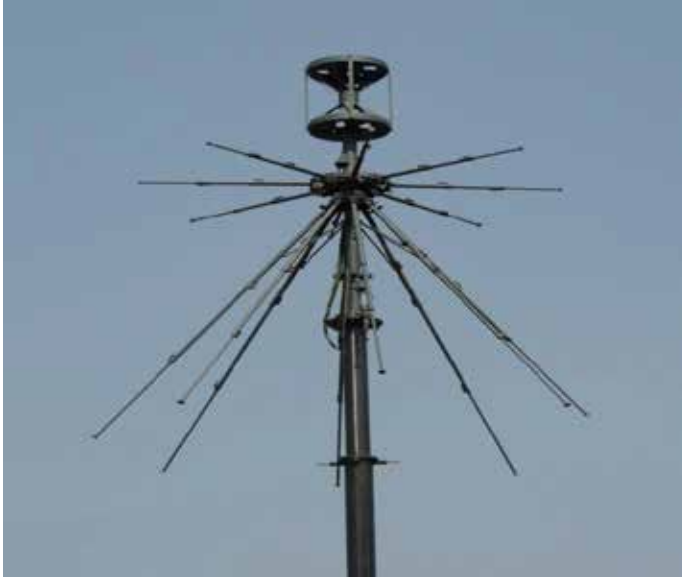
2-bay Monitoring Antenna Sub-system
