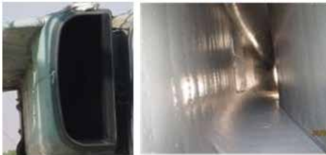
RAP Application inside Air Intake Duct
