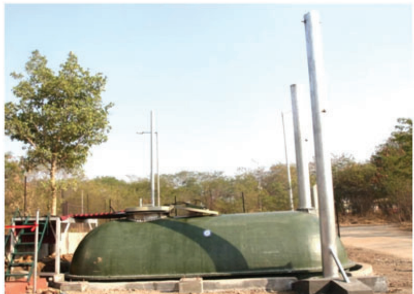
Composite underground shelter
