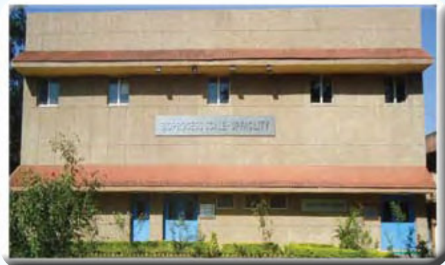
Bioprocess Scale-up Facility
