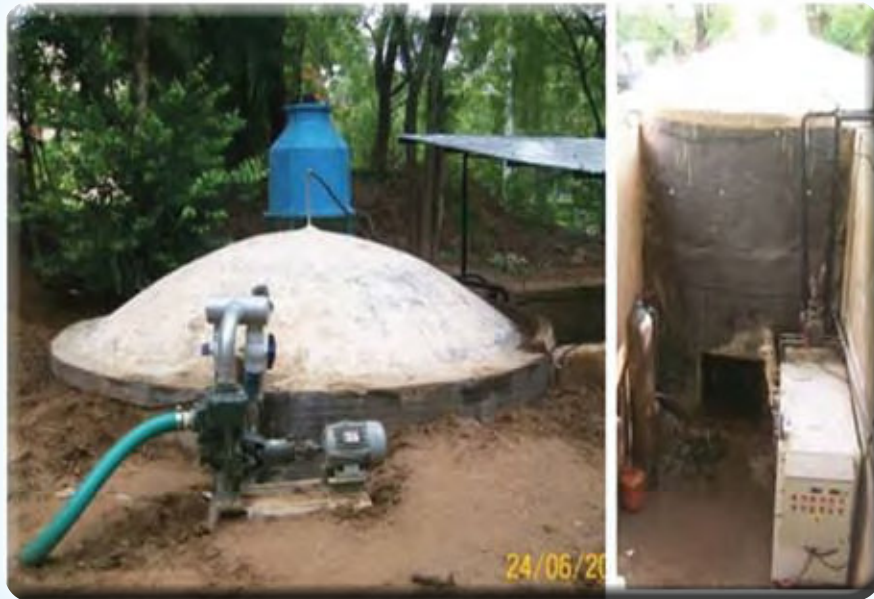
Anaerobic Microbial Inoculum Generation Facilities of 14 m 3 and 70 m 3 at DRDE
