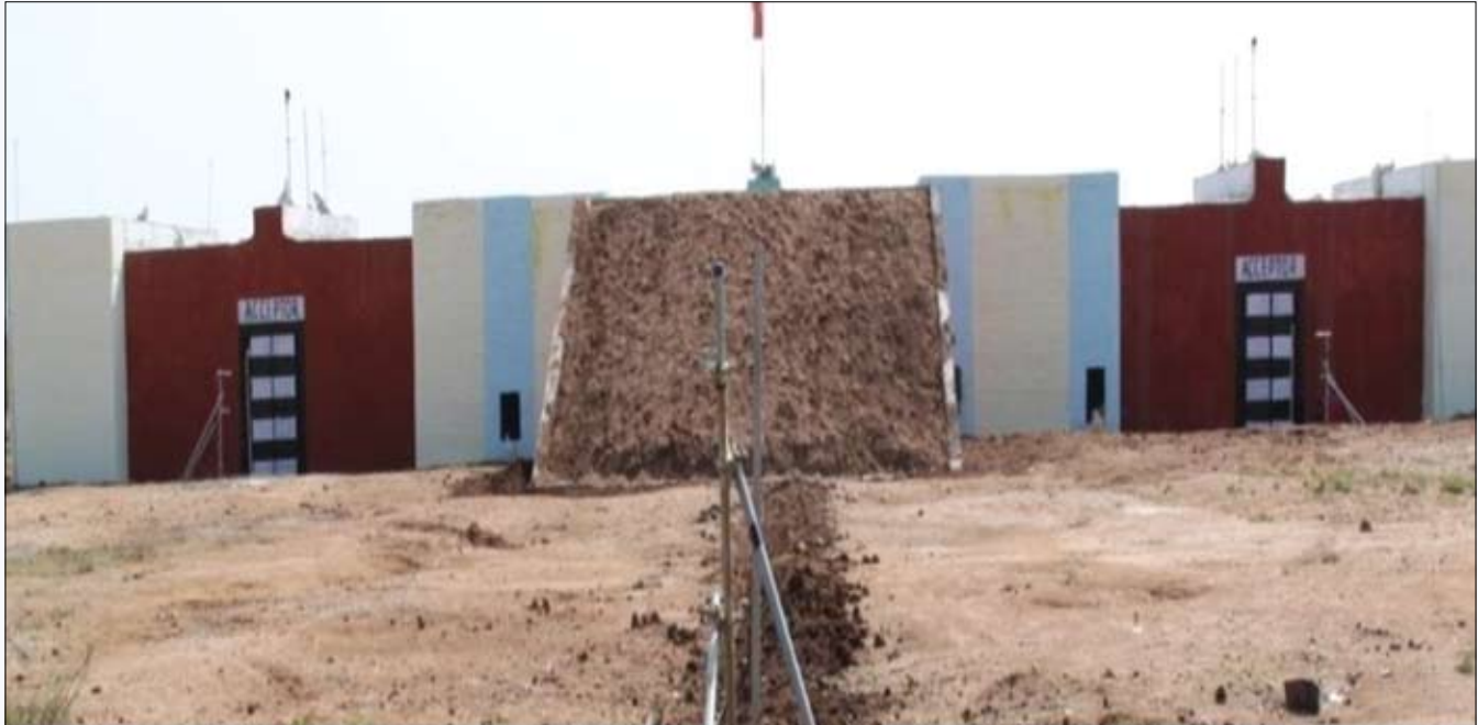
High Performance Magazine Structure with Blast Gauges
