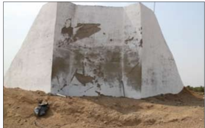
Portal Barricade After Explosion at Adit of UG Structure
