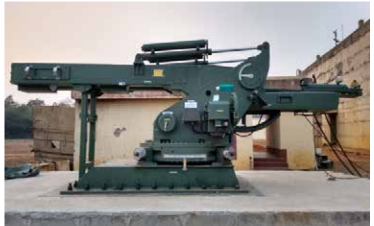
Installation on Grouting Platform at PXE, Balasore
